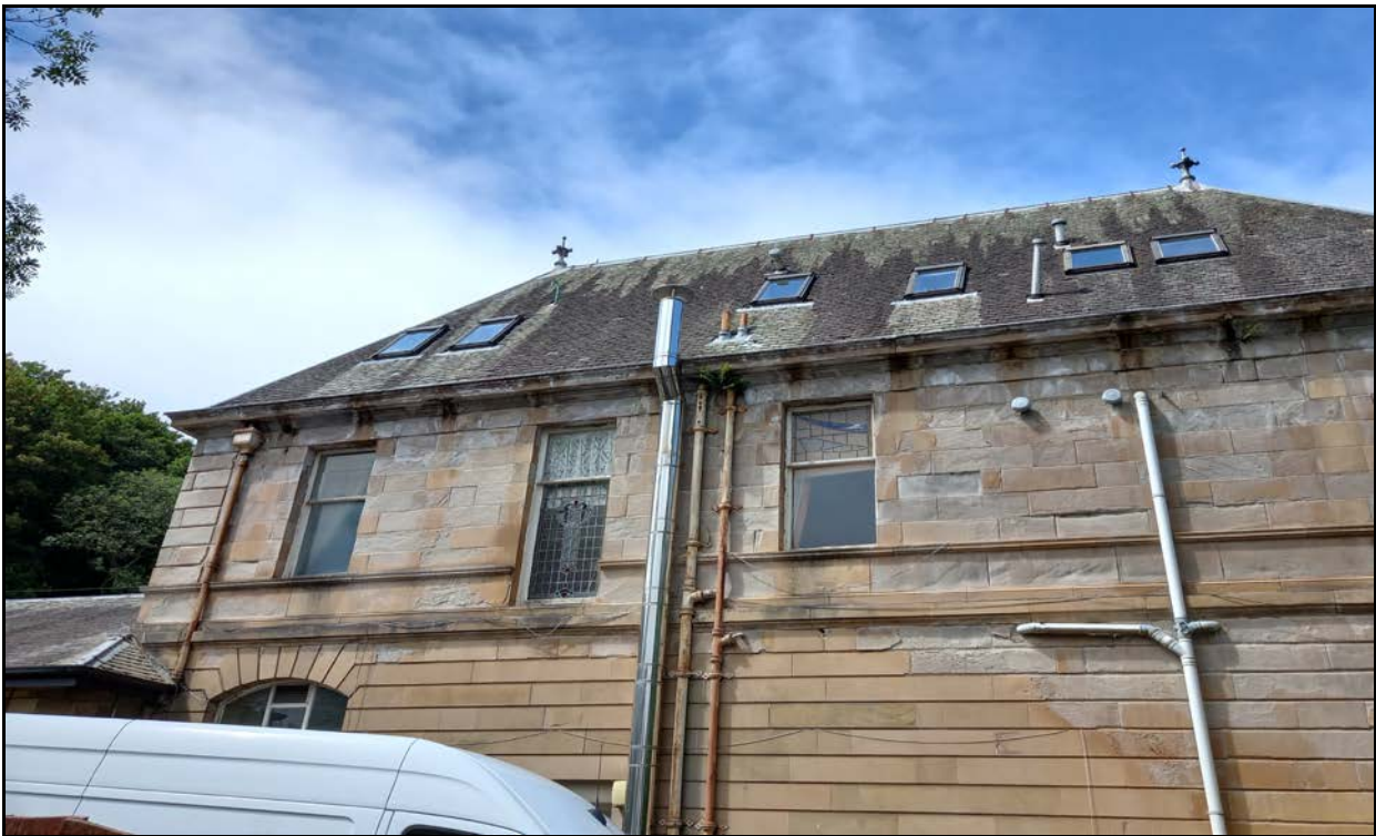
View of side elevation of the building
