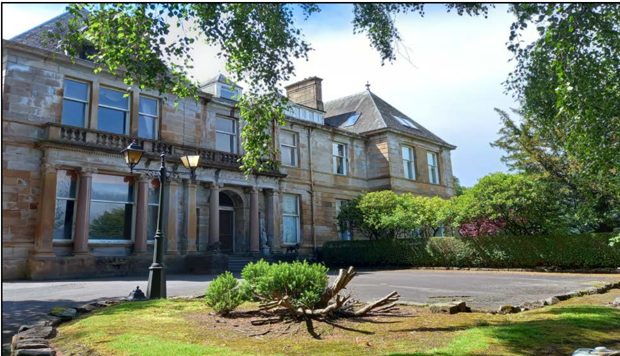
View of front elevation of the building
